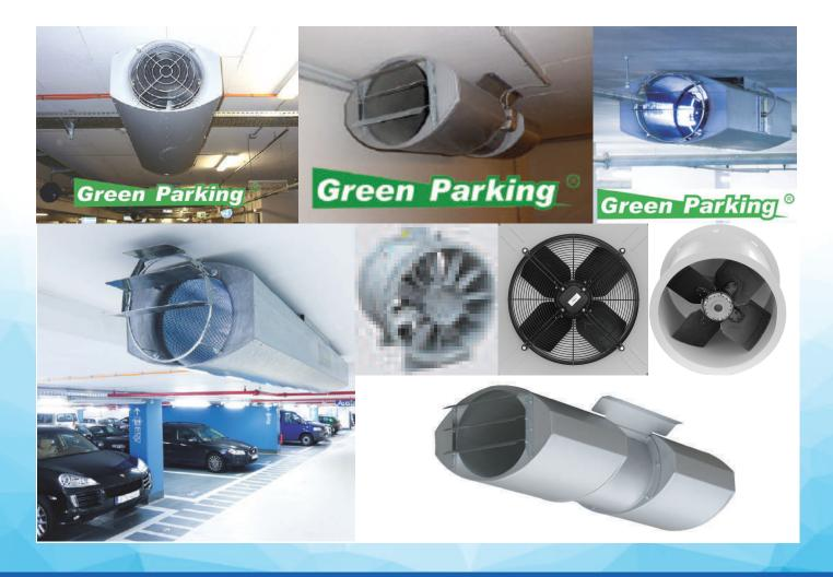
Burprovent has developed car parking ventilation system using Impulse type Jet fans and is heading the design team of Burprovent. They have adopted tunnel ventilation methods to car park ventilation systems & proved the system. This Car parking system is an intelligent system where the operation of the Jet fans, main extract & supply fans are controlled by CO & Fire detectionsystems.
